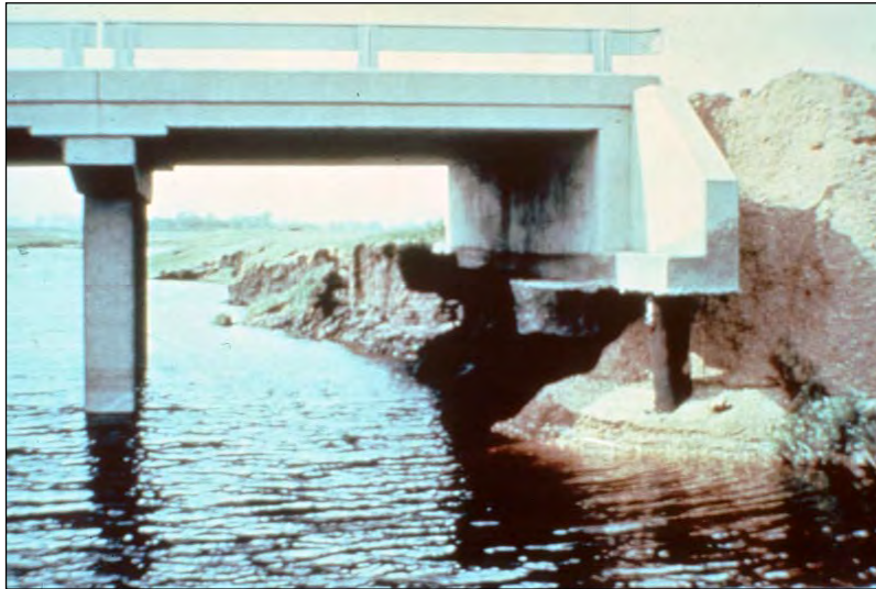
Figure 8.2. Scour of bridge abutment and approach embankment.
