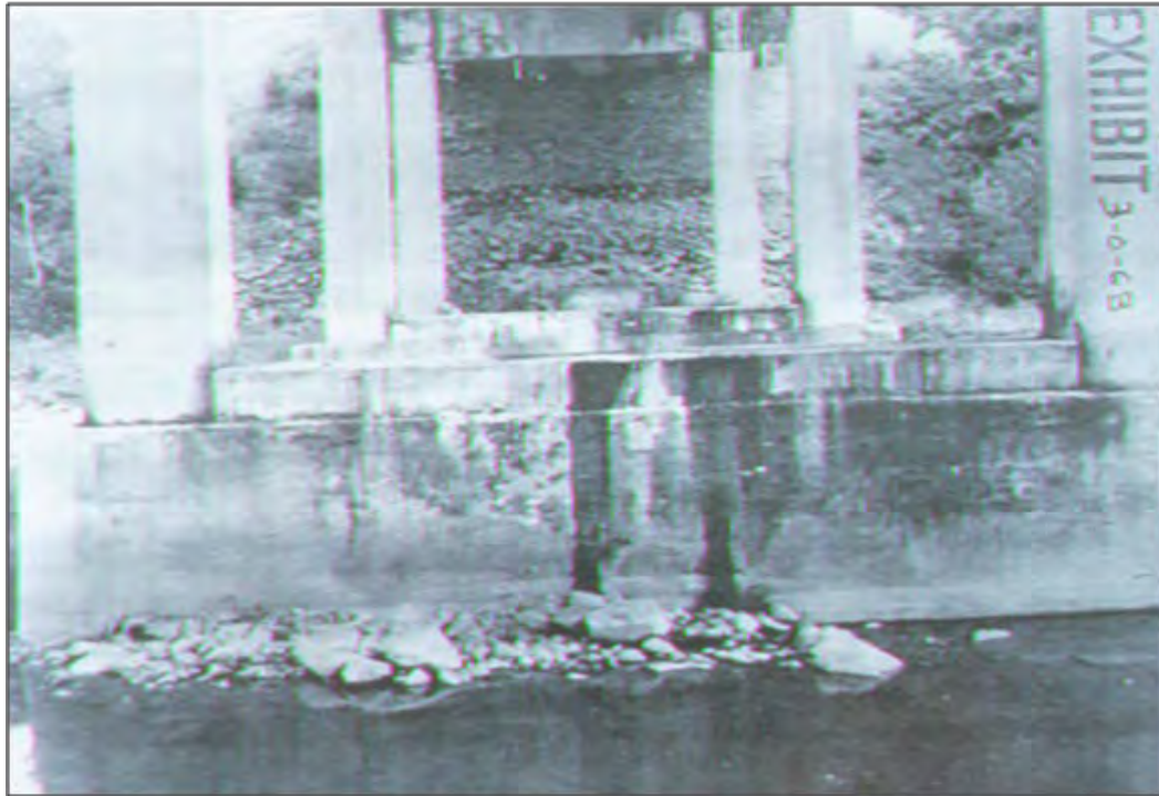
Figure 10.2. Photograph of riprap at pier 2, August 1977 (flow is from right to left).
